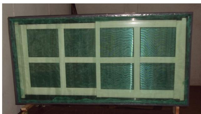
**Figure 2.** Inverted S/O channel/grip window frame (ISOWF) with hoisted net and housing aluminium window slide shutters (anterior view, note the greenish tinge due to the colour of the mosquito net).
